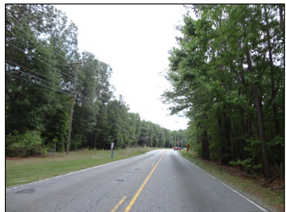
Miles Jamison Road facing east (site on the right)
